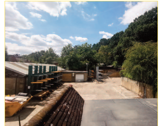
Rear view of 66 Brox Road
